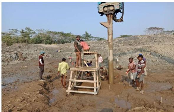
Figure 3-66: Executing the Sand Pile For DS-5 of Polder-40/2
