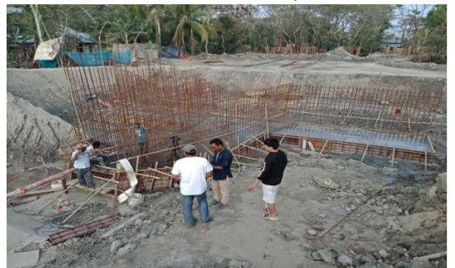
Figure 3-67: Fixing the Deformed Bar For FS-10 of Polder-40/2
