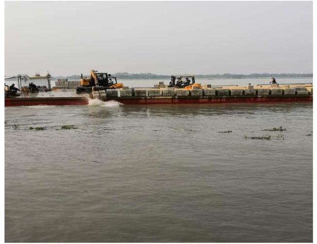
Figure 3-63: CC Blocks dumping for river bank protection work in Polder 39/2C
