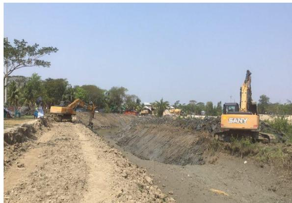
Figure 3-75: Excavating the Drainage Channel Near DS-3-4 of Polder-47/2
