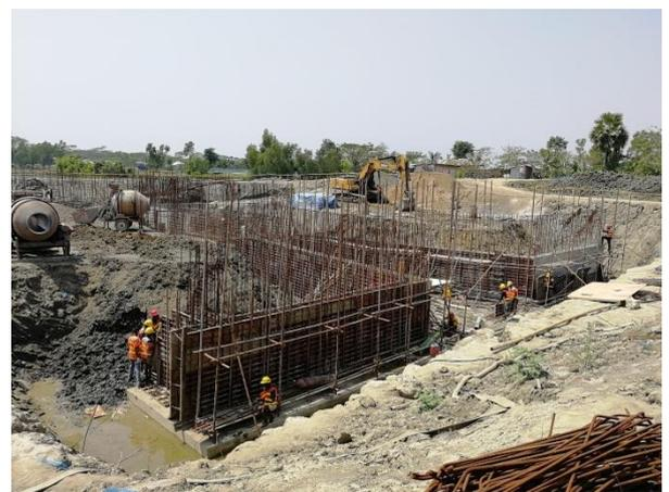
Figure 3-73: Establishing the Form for RCC Wall for DS-3 of Polder-47/2
