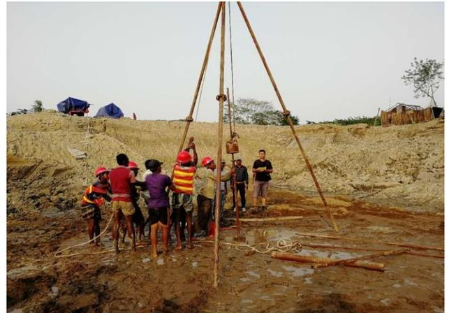
Figure 3-65: Drilling the Dewatering Bore Hole For DS-5 of Polder-40/2
