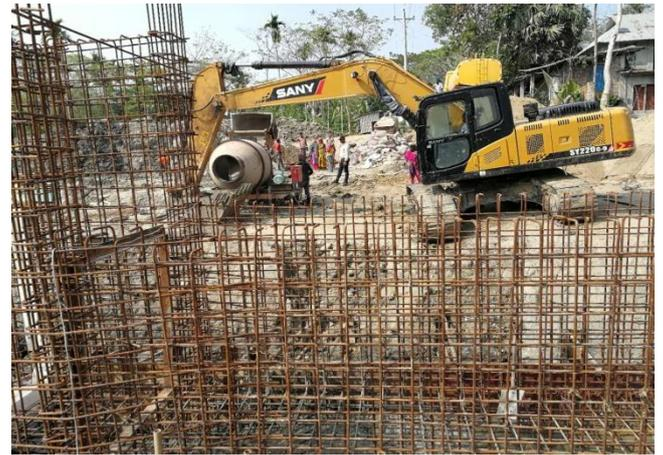
Figure 3-69: Pouring the RCC Box Base Slab For DS-9 of Polder-41
