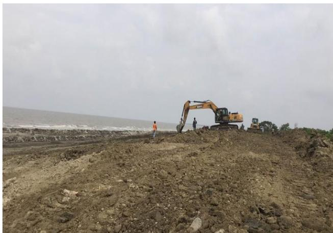
Figure 3-74: Construction of EMB Near K34+600 of Polder-48
