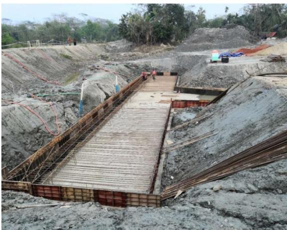
Figure 3-72: Establishing the LC form for DS-7 of Polder-43/2C
