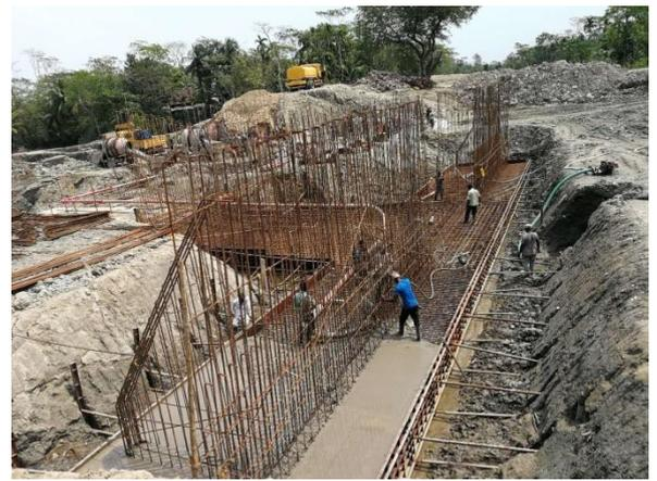
Figure 3-71: Pouring the RCC Base Slab For DS-6 of Polder-41/1
