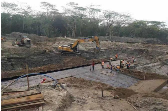
Figure 3-64: Pouring the Lean Concrete For DS-7 of Polder-39/2C
