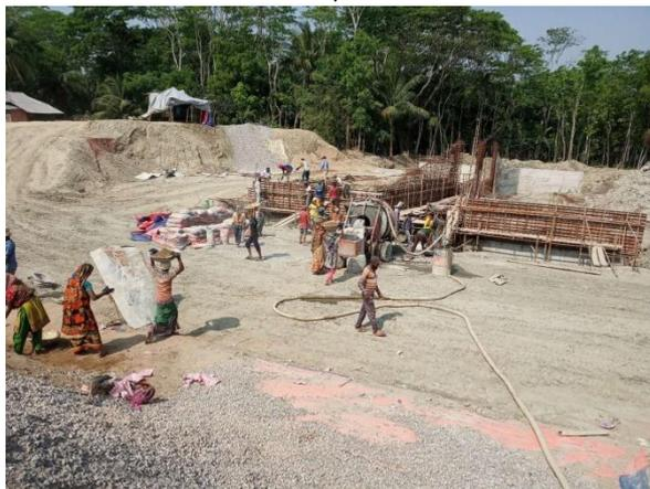
Figure 3-70: Pouring the RCC Wall for FS-1 of Polder-41/1
