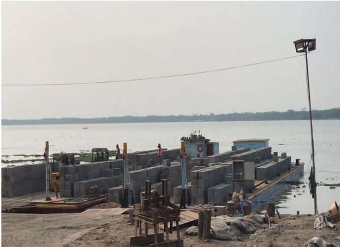
Figure 3-62: Loading The CC Block For River Protection Works of Polder-39/2C
